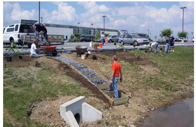
Installation of the water ladder for runoff erosion control
