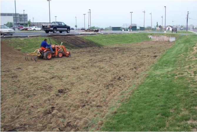
Plowing the east basin floor before sowing the area with meadow grasses and forbs
