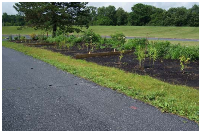
Newly planted rain garden; note wooden baffles. Additional plants were added in the Fall of 2006
