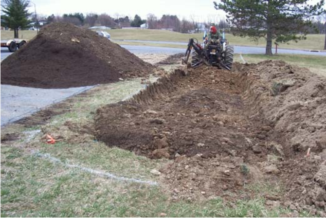
Excavation of the bioretention cell, early Spring 2006
