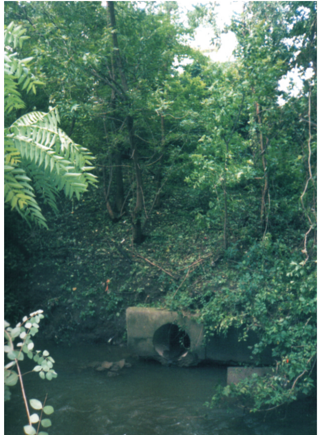
Combined Sewer Outlet
